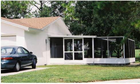
Unacceptable: prefabricated screen room.
