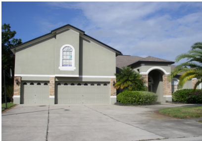
Unacceptable: "lopsided" upper floor on one side
