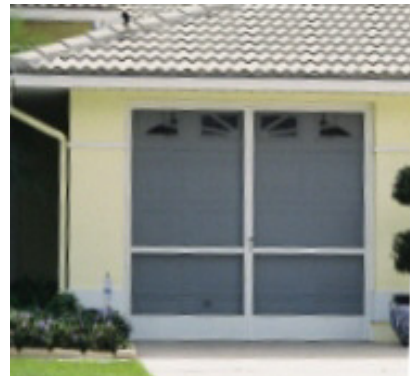
Unacceptable: screened in over garage
