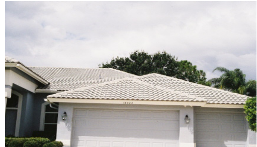
Acceptable: barrel tile or "S" tile roofing
