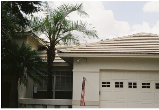
Acceptable: flat tile roofing
