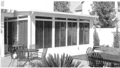
Unacceptable: Flat roof sunroom
